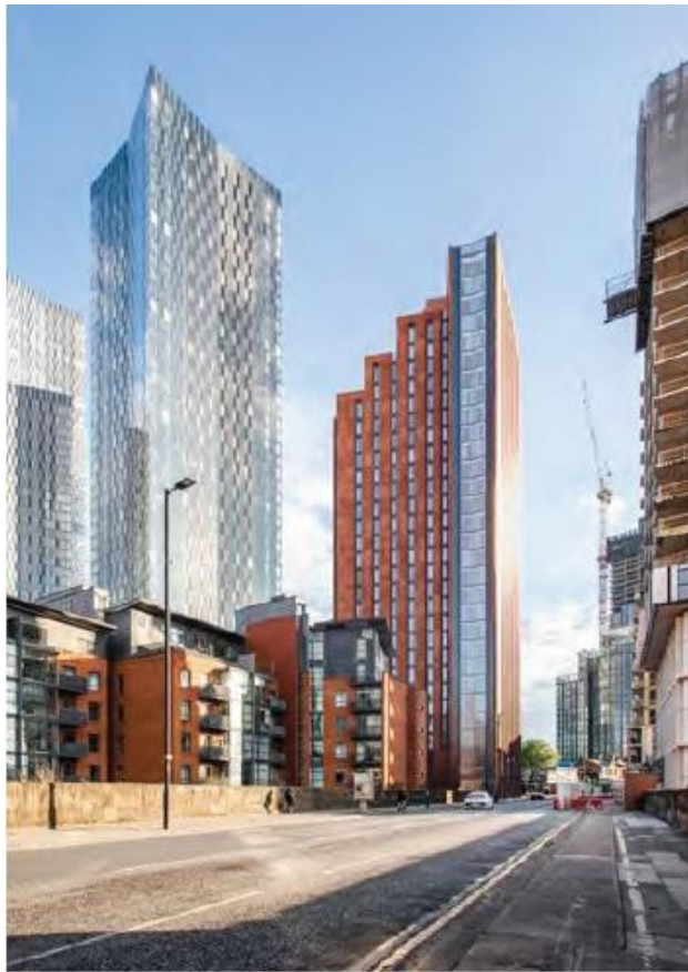
View from North-Eastern approach along Bridgewater Viaduct
